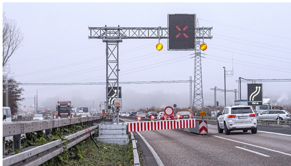
Intelligent alternating traffic management from Zeppelin Rental: Digitally controlled traffic management reduces traffic congestion and lowers CO 2 emissions at construction sites
