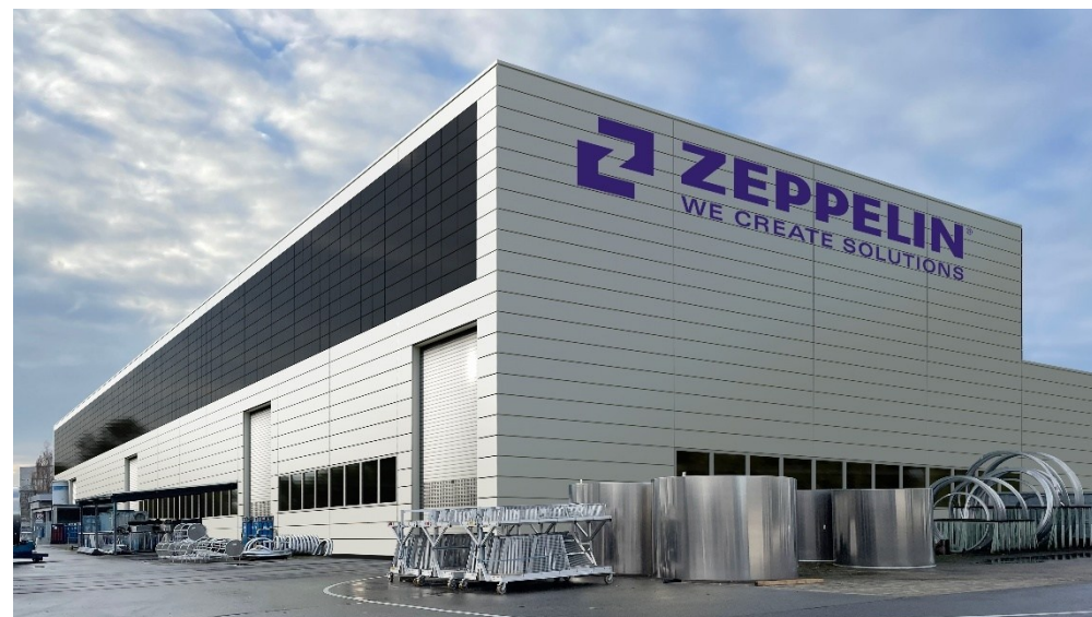
Ludwig-Dürr production hall in Friedrichshafen: A facade-integrated photovoltaic system with 1,280 glass-on-glass modules contributes to the energy-efficient building envelope and supports the self-generation of electricity at Zeppelin System's plant engineering site
